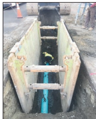
A 12-inch PVC Sewer Main installation, approximately 10 feet deep.
