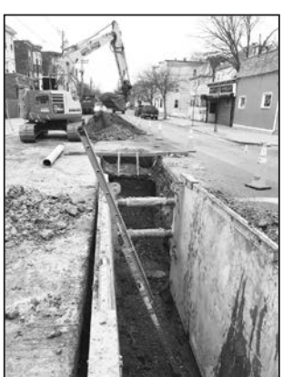
The contractor has to find unique ways to support existing utilities.
