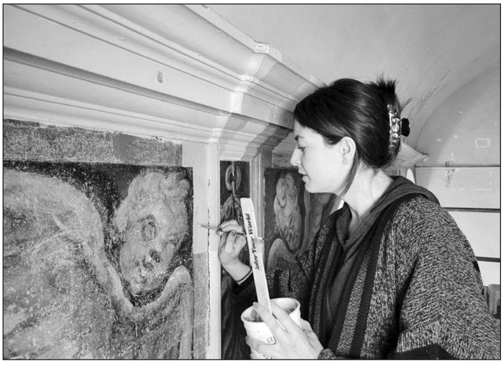
A worker painstakingly removes layers of white paint to partially uncover one of the angels painted in 1727.
